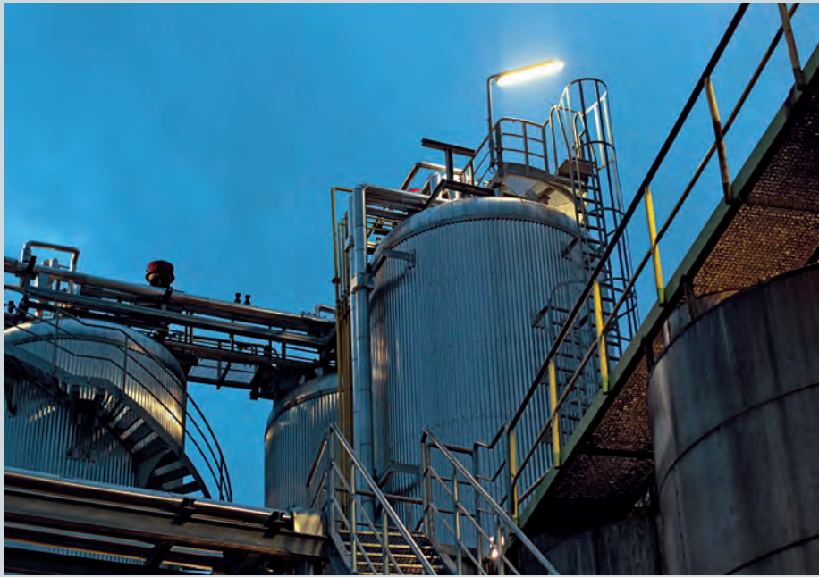
Our own large-scale tank farm allows for the intermediate storage of our core and by-products.
